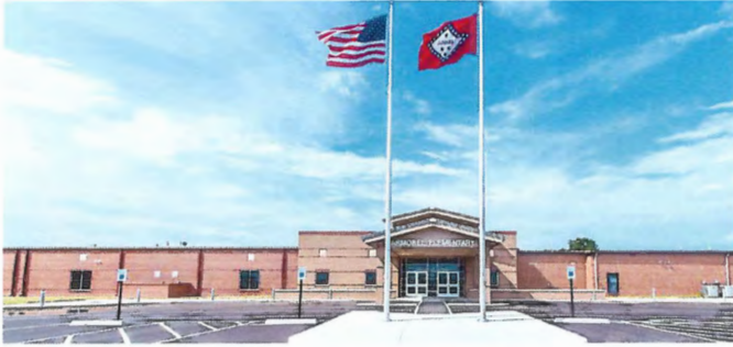
ARMOREL SCHOOL DISTRICT K-4 Building Addition & Renovations
