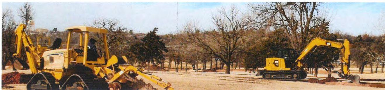
IRRIGATION INSTALL AND SHAPING EXCERSIZE SIDE-BY SIDE
